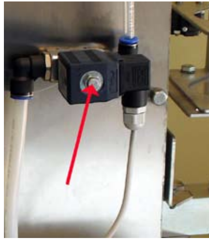
Fig. 7. P35 Solenoid Valve. Remove nut, casing, and then valve stem.
