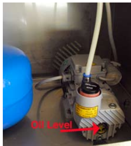
Fig. 6. P35 Vacuum Pump. Check oil level daily. Fill to mid-level in window.
